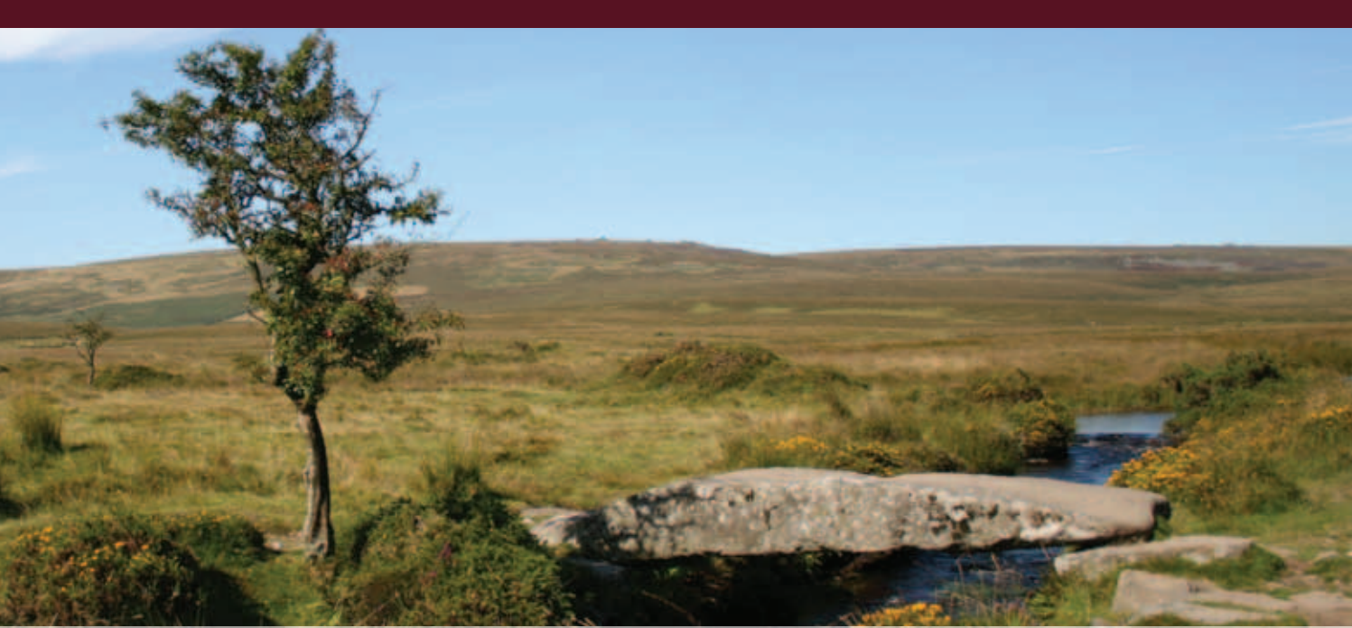
Wallabrook clapper bridge
